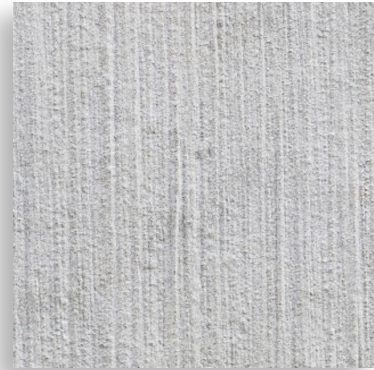
Tilt-Up Concrete Wall LIGHT BROOM FINISH
