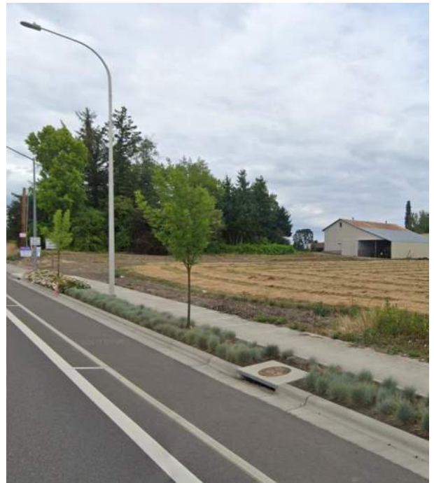
Example of separated pedestrian facilities on Brookwood Parkway in Washington County, OR
