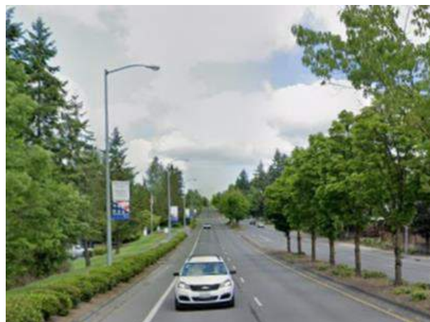
Typical roadway lighting along a multilane facility
