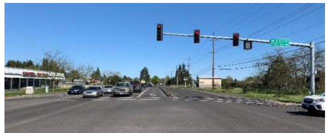
Eastbound permitted/protected left-turn display and low visibility of tubular markers
