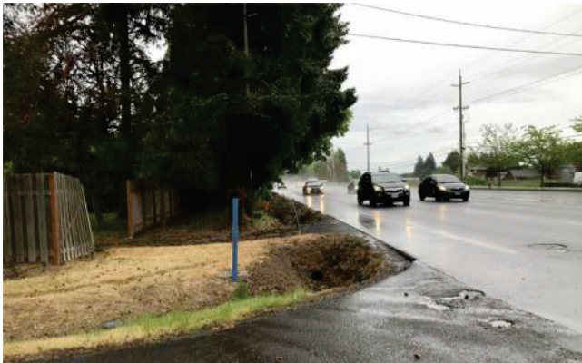
At 336 th Avenue looking east
