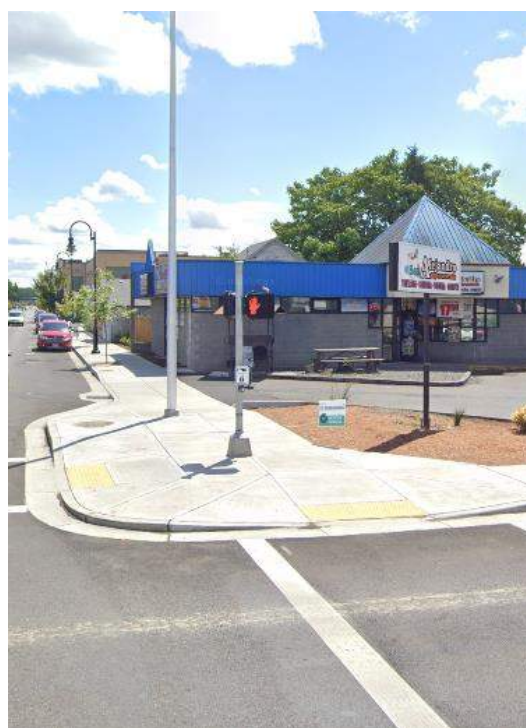
Illustration of ADA-Compliant Pedestrian Ramps
