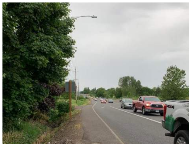
Lack of eastbound bike lane at 17 th Avenue
