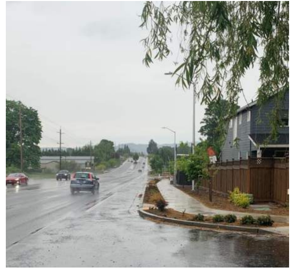
Example of Short Segment of Existing Lighting on the Corridor
