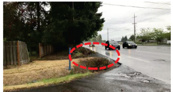
Driveway near 336 th Avenue
