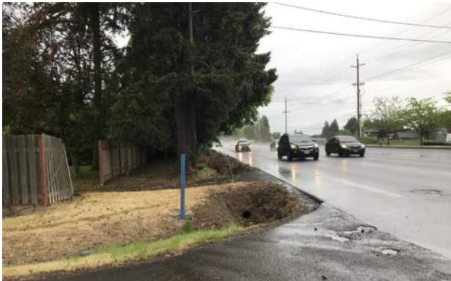
At 336 th Avenue looking east
