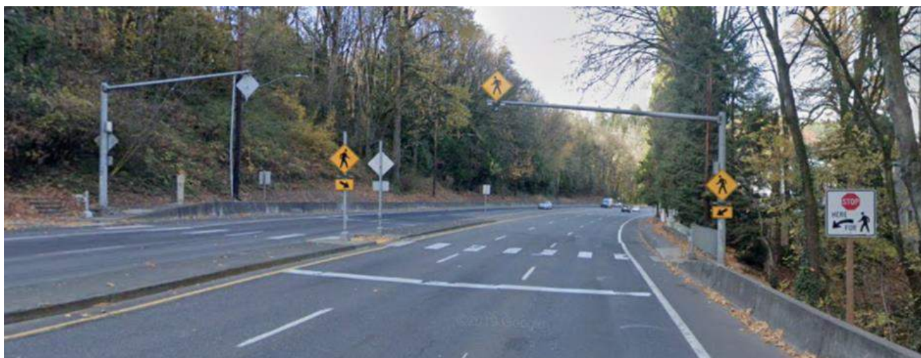
Example of Overhead RRFB Installation
