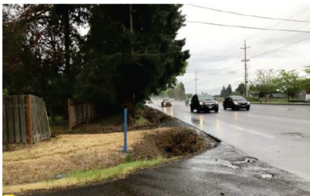
At 336 th Avenue looking east
