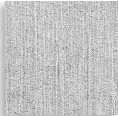
Tilt-Up Concrete Wall LIGHT BROOM FINISH
