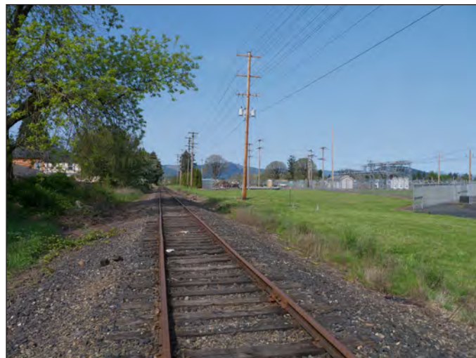
Rail corridor near BPA substation
