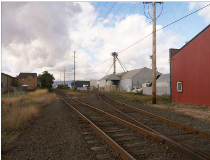
Rail siding west of N 10th Ave.
