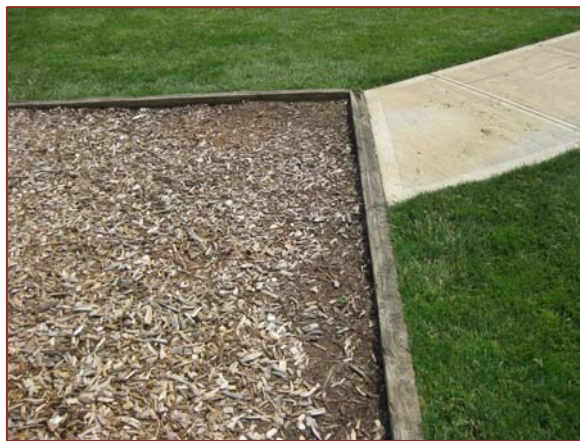
Figure 14. Playground access requires ramp for ADA compliance
