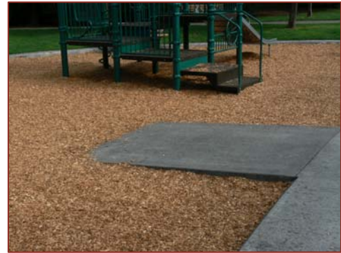
Figure 35. Example of ADA-compliant ramp into play area
