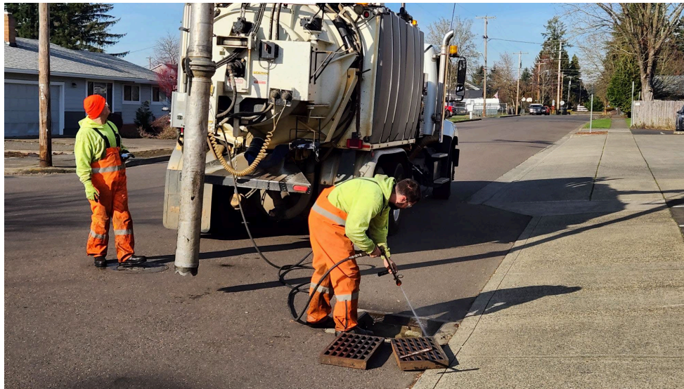
Staff cleaning a Storm Drain
