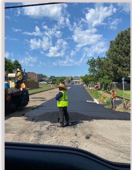
Repaving North Clark Street
