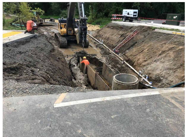
Laurel Woods Sanitary Sewer System Installation
