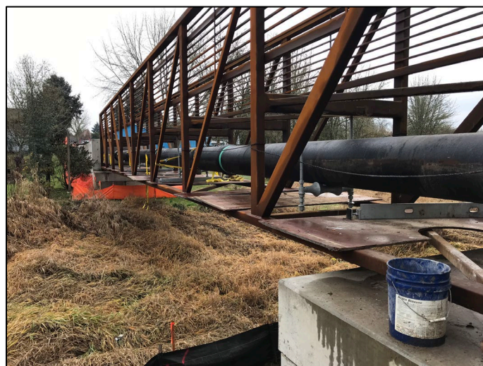
Ginger St. Sewer – East Bridge
