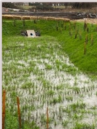
Laurel Woods Water Quality Facility
