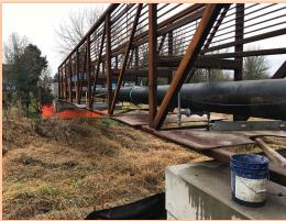
New bridge supporting sewer pipe carrying wastewater from SE quadrant of city to the treatment plant in Forest Grove. This pipe and bridge replace a 45-year old underground, high maintenance system.
