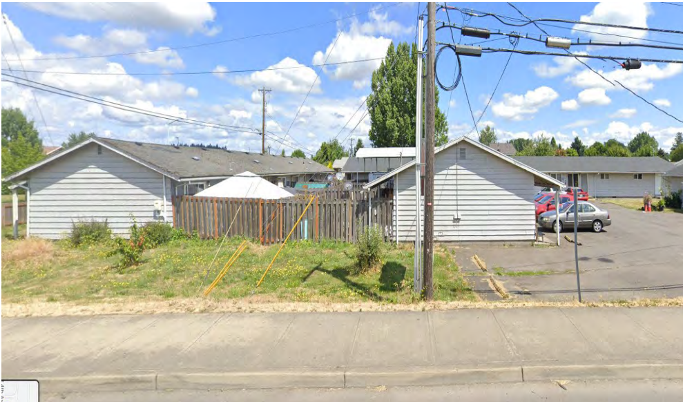
PHOTO 20 Apartments to the North across TV Highway.
