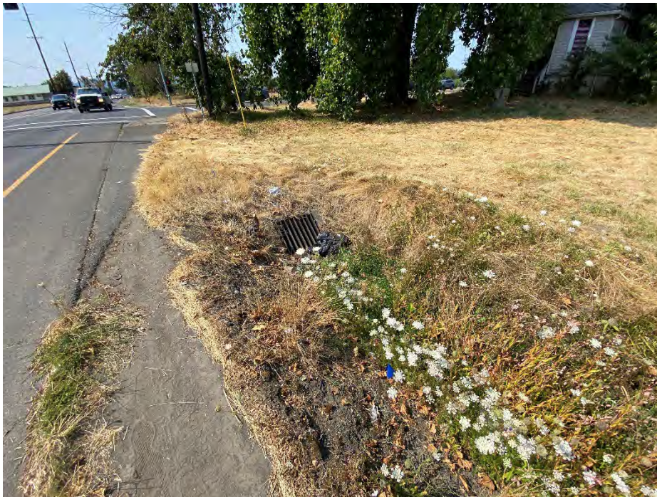
Photo 12 Storm drain South side of site.
