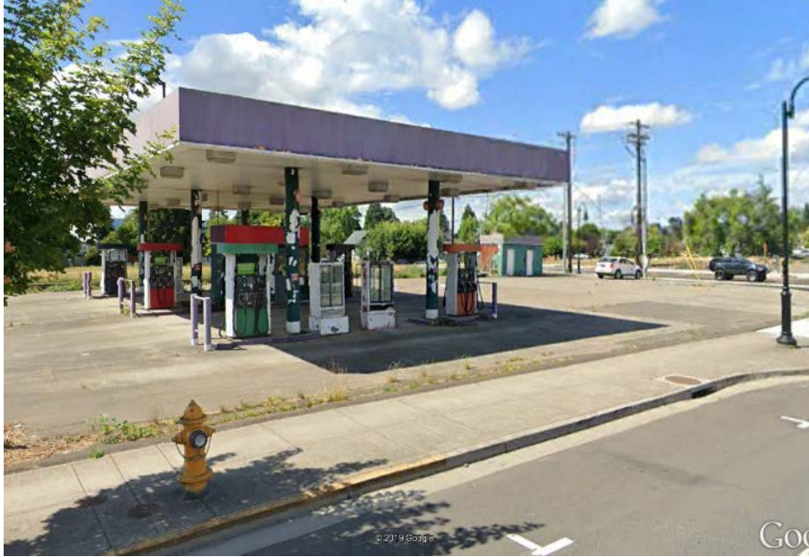
Blighted commercial property identified for City acquisition and cleanup
