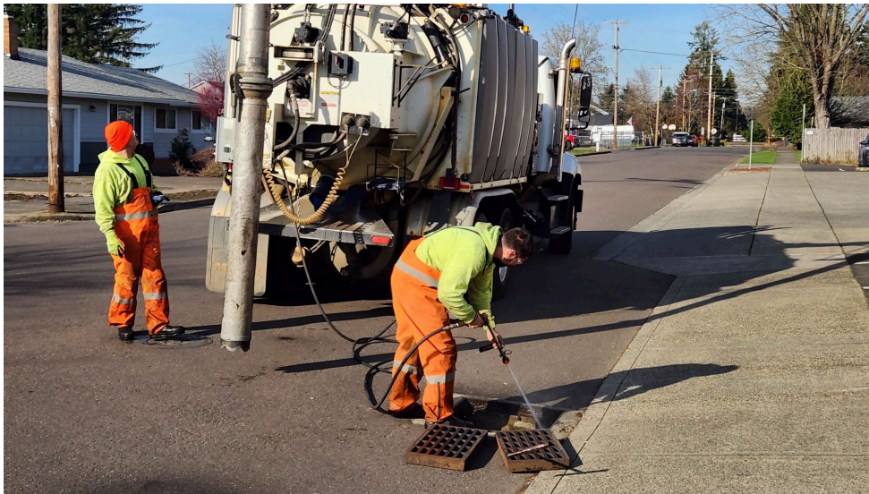
Staff cleaning a Storm Drain
