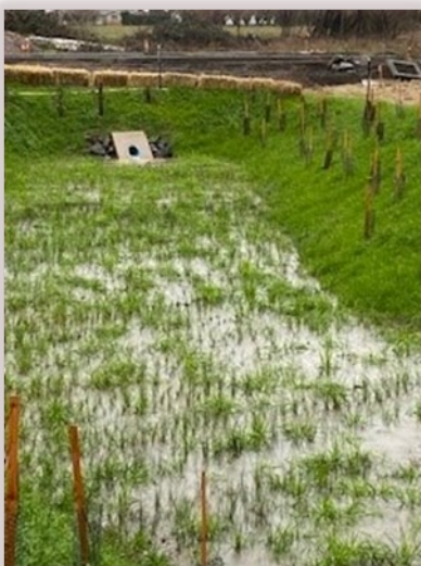
Laurel Woods Water Quality Facility
