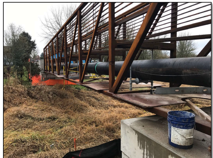
Ginger St. Sewer – East Bridge
