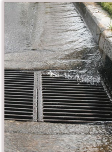
Catch Basin/Storm Drain
