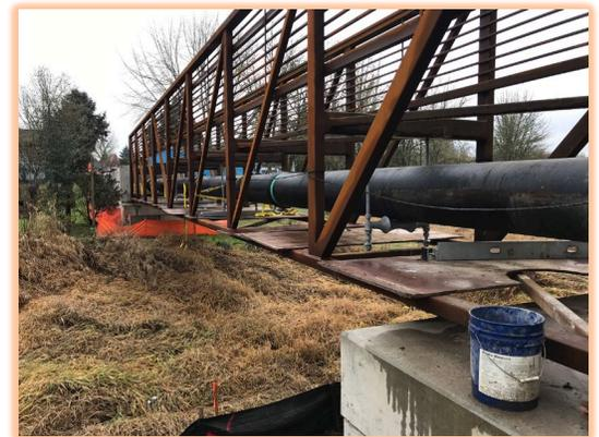
*New bridge supporting sewer pipe carrying wastewater from SE quadrant of city to the treatment plant in Forest Grove. This pipe and bridge replace a 45-year old underground, high maintenance system.*
